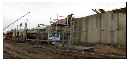
Kitchen, labs and classrooms taking shape
